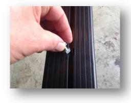
Locate all the legs, spacing them equally along the rack. Do not fully tighten at this stage.
